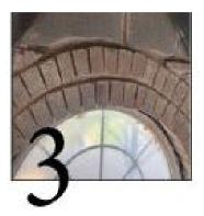
steel reinforcement rods were also installed behind the bricks located above the windows to prevent the bricks from moving apart (see pictures 1-6). Lastly, rustproof paint was applied to the metal support that is helping to hold the limestone in place at the louver level.
